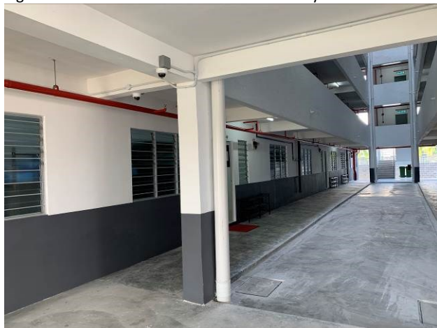
Figure 6: First floor corridor outside dormitory units
