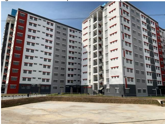
Figure 5: Two eleven-story blocks at Bukit Minyak CAT
