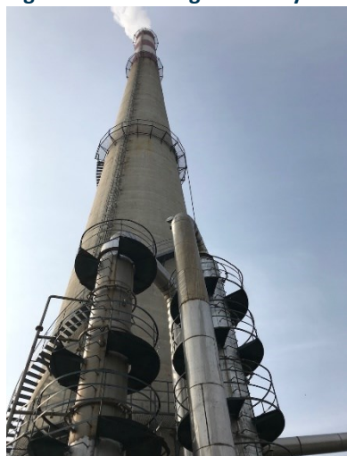
Figure 27: 120m high chimney to exhaust gas
