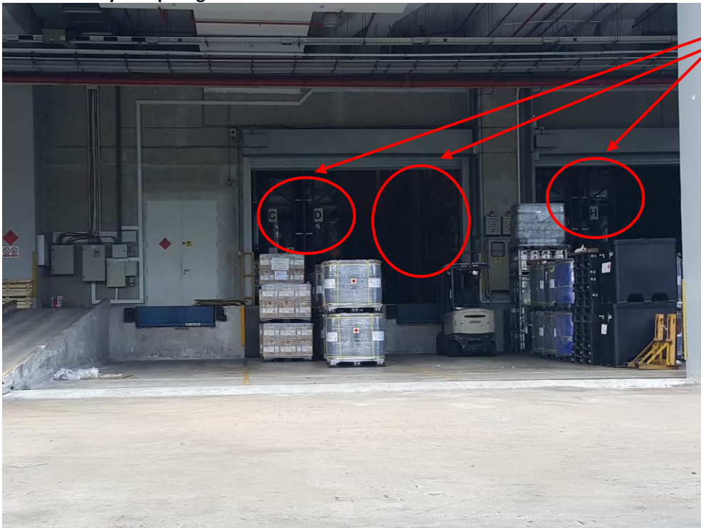
Exhibit 4. Fully occupied ground floor warehouse
