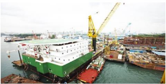
Construction of McDermott LB32 pipelay barge
