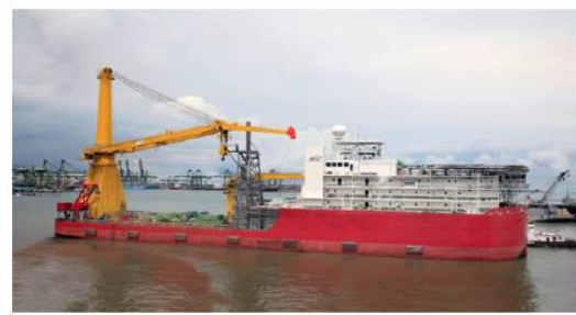
Retrofitting of Jascon 25 pipelay barge
