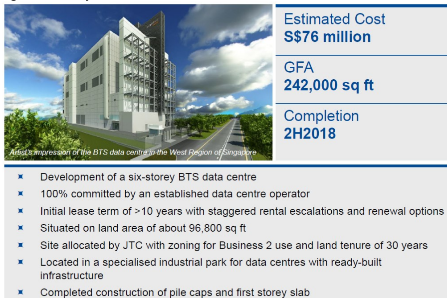
Figure 2: BTS Project – New Data Centre
