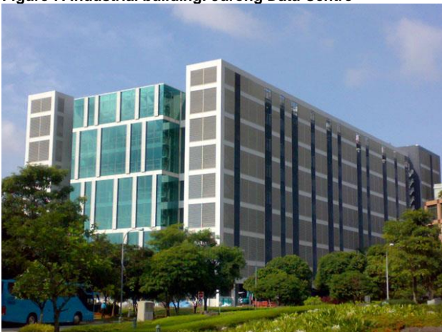
Figure 7. Industrial building: Jurong Data Centre
