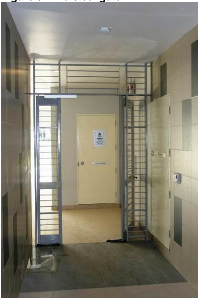
Figure 5. Mild steel gate
