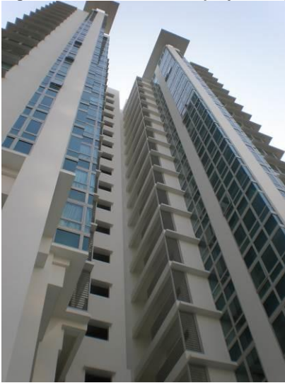
Figure 9. Private residential project: Meyer Residence
