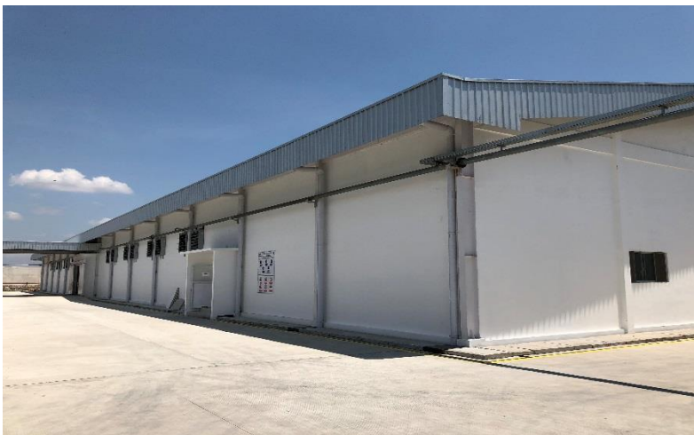
Figure 2: Outside one of many factory blocks
