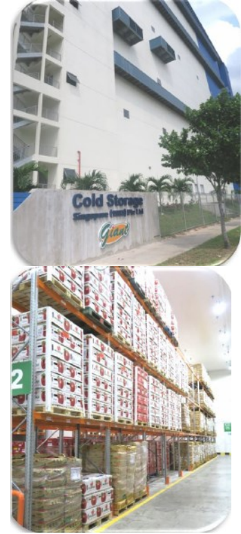
Figure 11 & 12: New Fresh DC in Singapore enables bulk handling
