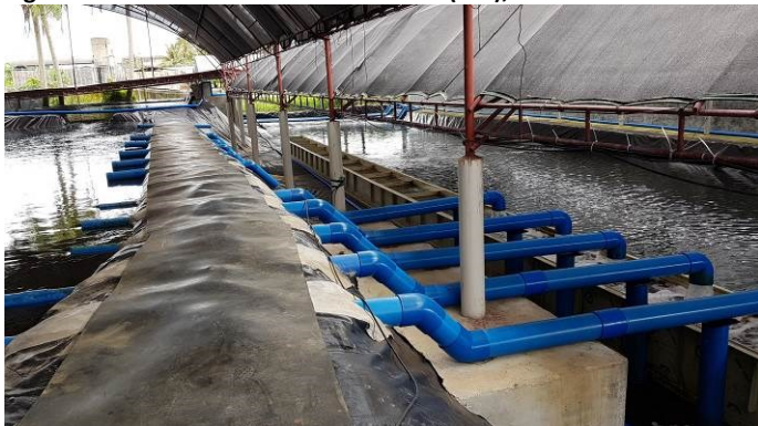
Figure 10: Sedimentation Ponds 1 and 2 (left), aeration and Treated seawater reservoir (right)
