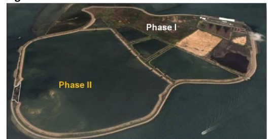
Fig 14. Aerial view of Phase I and Phase II
