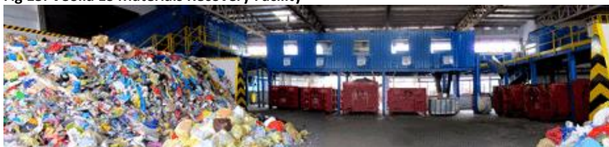
Fig 15. Veolia ES Materials Recovery Facility
