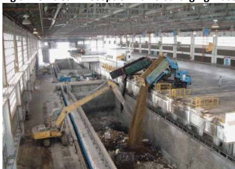
Fig 9. Vehicles in reception hall discharging waste directly onto the barge
