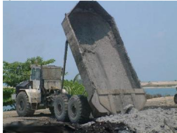
Fig 13. Dump truck unloading incinerated ash at landfill cell
