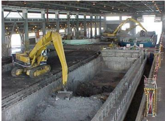
Fig 12. Excavators removing waste from barge
