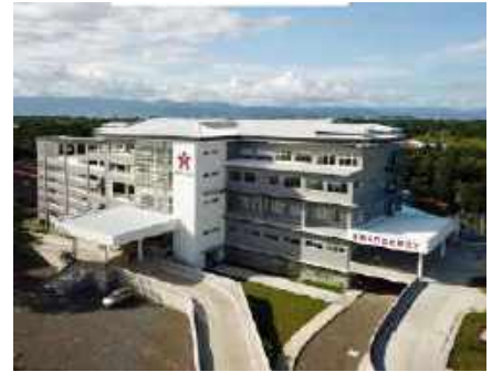
Figure 13: One branch inside a hospital in Lapulapu City, City
