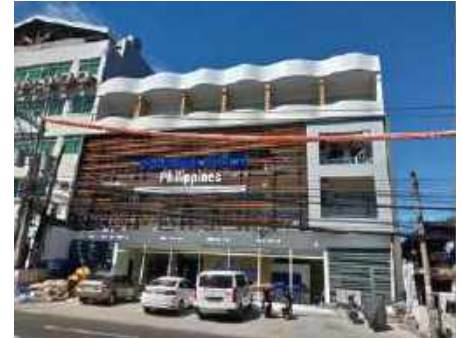
Figure 9: The 4-storey medical centre
