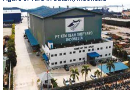
Figure 6: Yard in Batam, Indonesia
