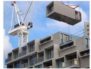
Figure 17: PPVC module installation
