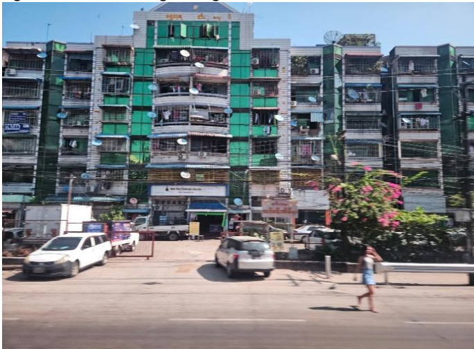
Figure 11: Older housing in Yangon
