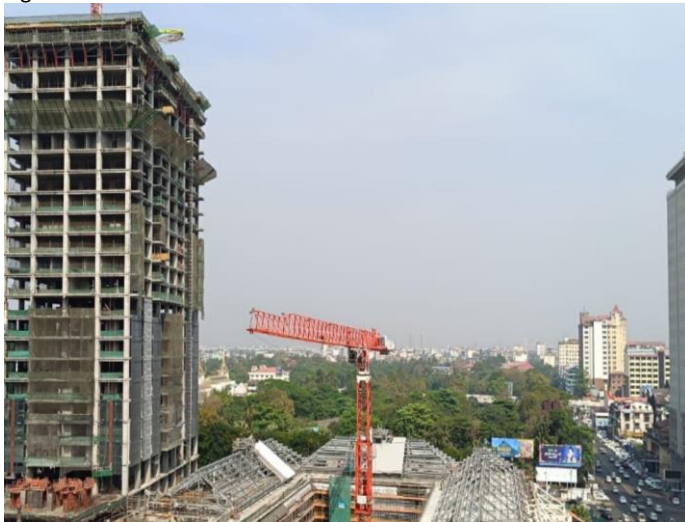
Figure 15: Yoma Central construction site
